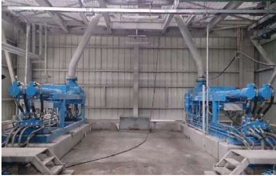
ABEL SH for mine backfilling at an altitude of 4800 m
